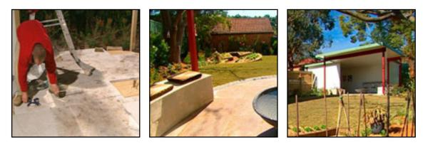
**Herb garden:** Jamie constructed a circular herb and vegetable garden and because it was on a slope, it had to be built up on one side. Jamie used ACQ pine sleepers and we cut these into large brick sizes to more easily create curves. A path was built through the circular garden to provide easy access to the herbs and vegetables.
