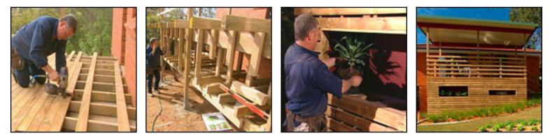
**Outdoor entertaining room:** We constructed a retaining wall from treated pine sleepers and then prepared the concrete slab for our outdoor entertaining area. We used sand to give the level for the concrete slab, followed by a plastic damp barrier and then the reinforcing mesh was laid on chairs. It was formed up with cut down form ply ready for concrete pour. We added black oxide to the concrete to give a charcoal look.
