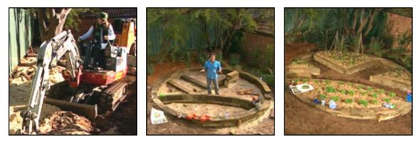
**ACQ Treated Timber:** Ammonium copper quaternary (ACQ) is an arsenic and chromium free preservative treatment and is one of the main types of timber preservative treatments protecting against fungal and insect attack. It is used for outdoor applications where below ground borer and rot resistant timber is required. Like other preservative treatments, it is essential to treat cut surfaces.
